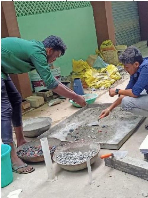
Figure 5.15: Prepration of Concrete
